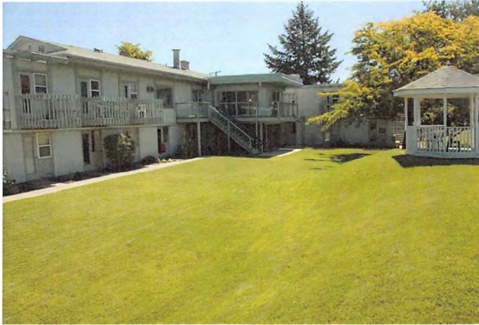
Photo 3. Typical landscaping at rear of subject property inside dike fence.
