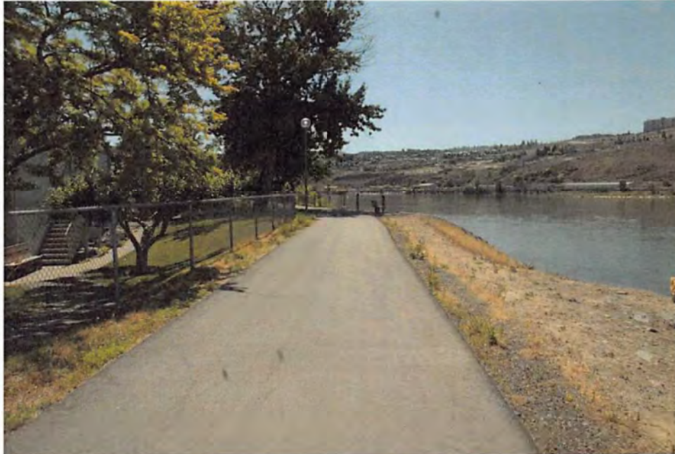
Photo 5. Paved dike crest behind subject property with limited vegetation and low potential for additional.
