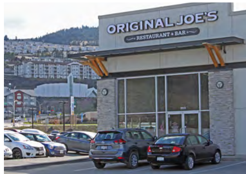
Entrances defined through features such as signage, awnings, and building materials can assist with public wayfinding
