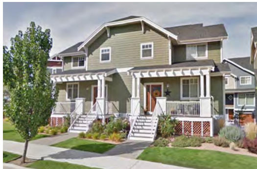
Paved pathways connect building entrances to the street, while comprehensive landscaping of front yards improves street appeal
