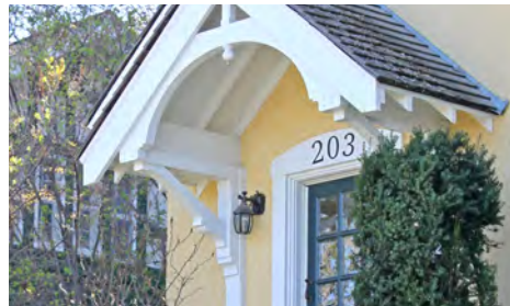
Example of high-visibility addressing with contrasting colours, lighting installed for illumination, and a covered entryway.
