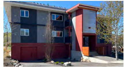
Narrow driveways separated by landscaping improve the street appeal of the development
