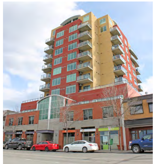
A podium set at the same height as abutting buildings help transition from shorter to taller buildings
