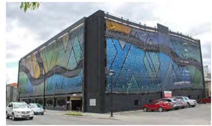
Structured parking on Lansdowne Street is screened by public art (work by Bill Frymire)
