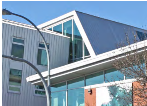
Making use of natural daylight in roof design can help reduce a building's energy consumption needs
