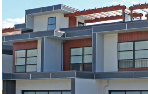
Offsetting windows from facing residential units and using window blinkers can help promote privacy
