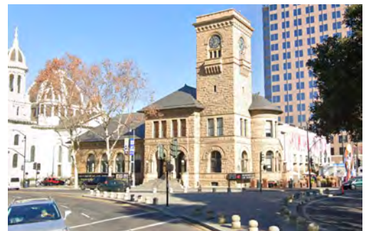
A clock tower creates strong definition at the street corner
