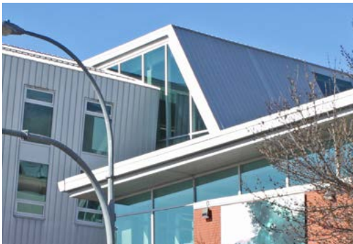
Making use of natural daylight in roof design can help reduce a building's energy consumption needs
