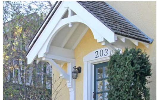
Example of high-visibility addressing with contrasting colours, lighting installed for illumination, and a covered entryway.
