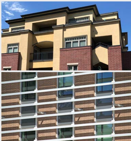
Deeper façades (recessed balconies) and window screens (louvres) along south- and west-facing building aspects protect residents from summer heat
