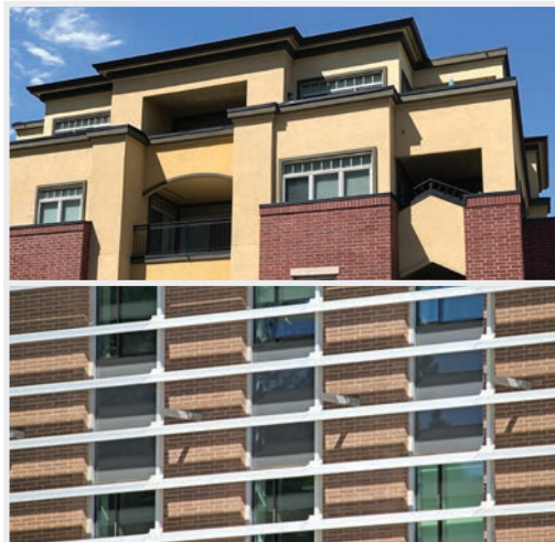
Deeper façades (recessed balconies) and window screens (louvers) along south- and west-facing building aspects protect residents from summer heat
