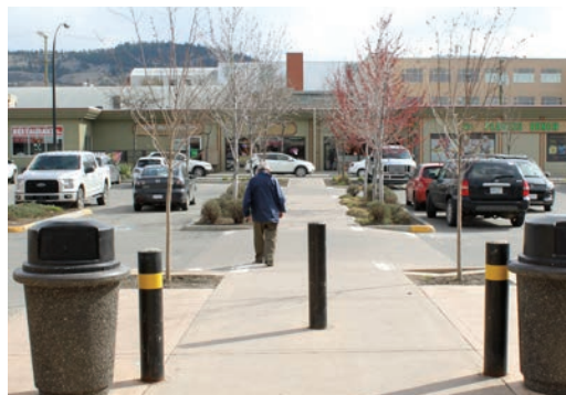
Raised pedestrian path through a commercial parking lot
