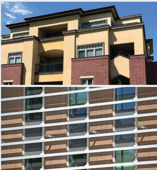
Deeper façades (recessed balconies) and window screens (louvers) along south- and west-facing building aspects protect residents from summer heat
