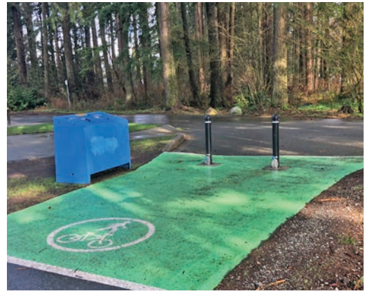
Permeable barriers, distinct material treatments, and street furniture help define use in public spaces and announce transitions
