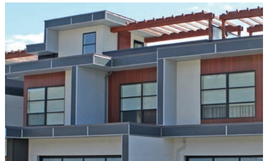
Offsetting windows from facing residential units and using window blinkers can help promote privacy
