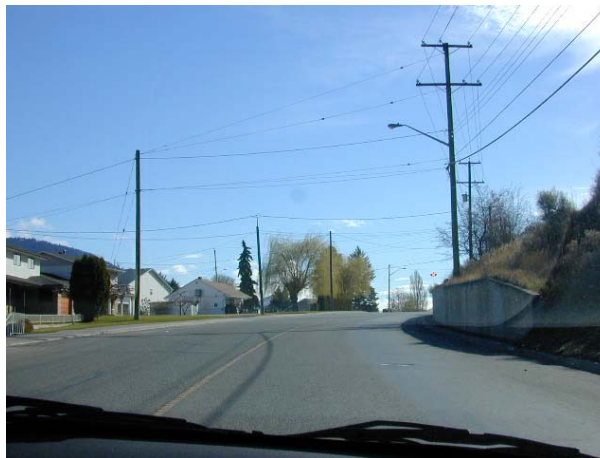
Curved approach and retaining wall reduces driver's view of the intersection, and of cross-street traffic.
