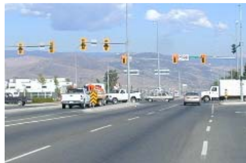
Example of an intersection with (good) signal visibility that exceeds the current policy
