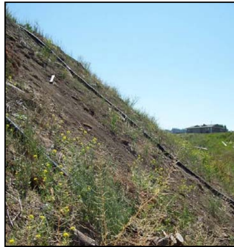
Steep slopes present a challenge for erosion control
