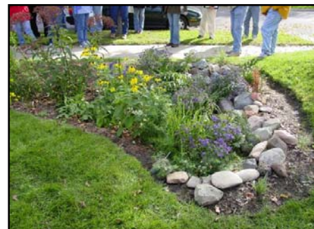
Example of a rain garden used for stormwater volume and quality control
