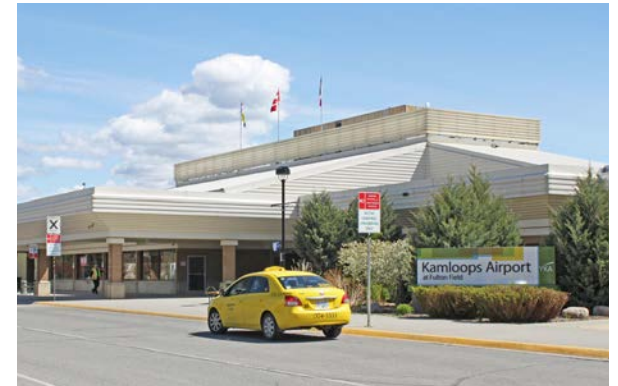
Air terminal building at Kamloops Airport
