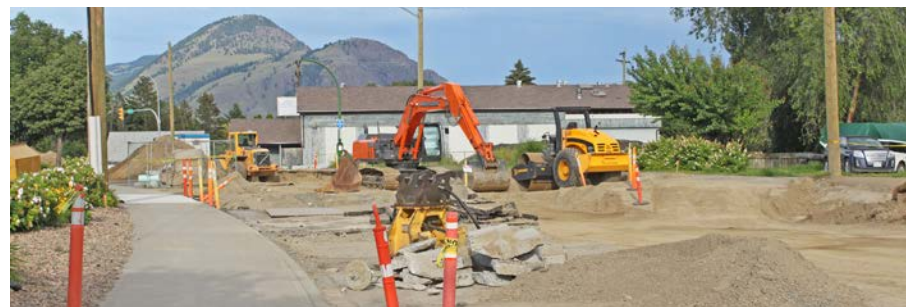
Phase 2 of the Tranquille Sanitary Main Upgrade under construction in 2020
