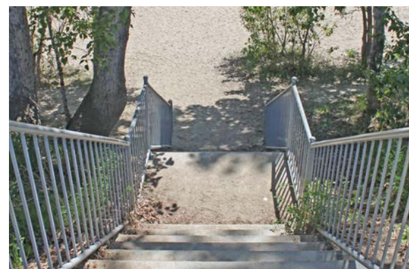
Stairway access at Overlander Park Beach
