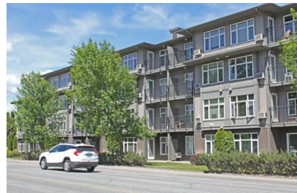
Multi-family infill housing along Fortune Drive
