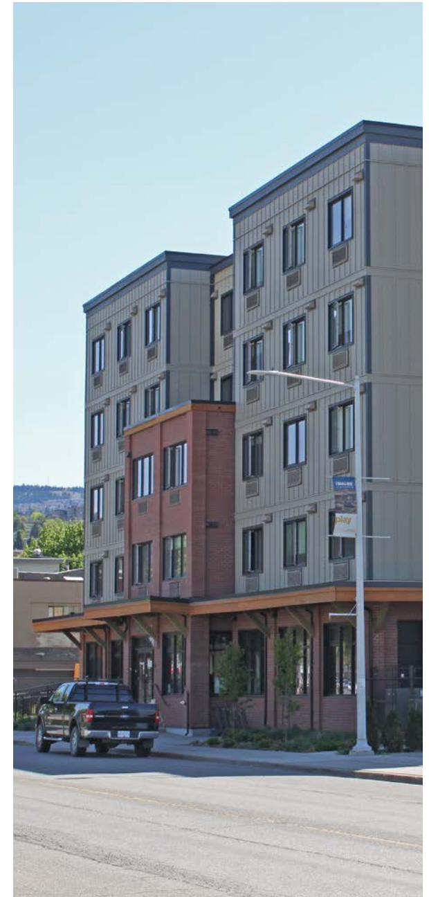
Spero House supportive housing on Tranquille Road
