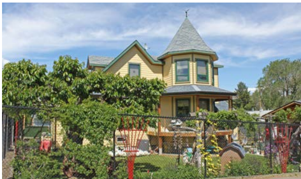
A house with heritage value on Nelson Avenue
