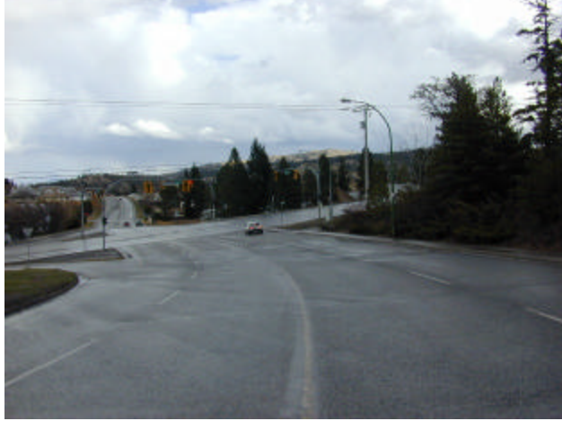
FIGURE G-3 CURVED APPROACH MEANS THAT SIGNAL HEADS ARE TO THE DRIVER'S LEFT, BLOCKED BY OTHER SIGNALS AND LESS VISIBLE UNTIL THE LAST MINUTE
