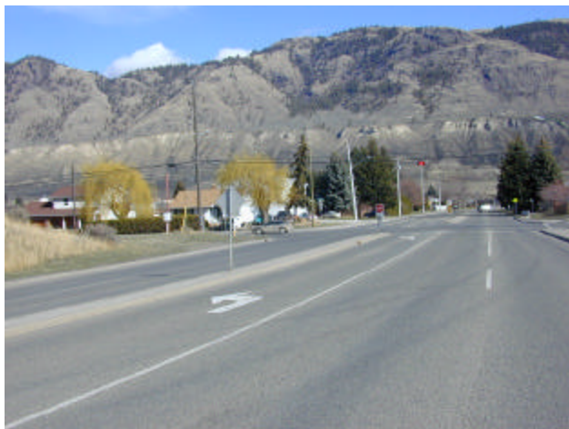
FIGURE G-5 MULTIPLE APPROACH LANES MEAN THAT DRIVERS MAY HAVE DIFFICULTY REMEMBERING WHO HAS THE RIGHT-OF-WAY
