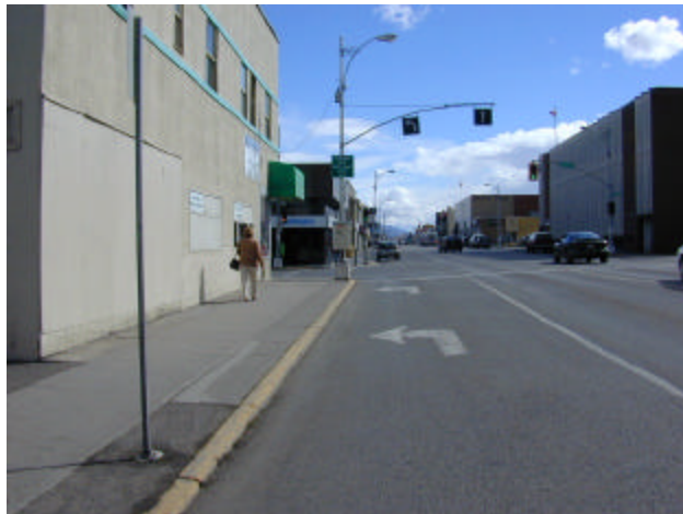
FIGURE G-1 PRIMARY SIGNAL HEAD OUTSIDE OF DRIVER'S CONE OF VISION (Also note how secondary signal head blends into buildings in the background.)
