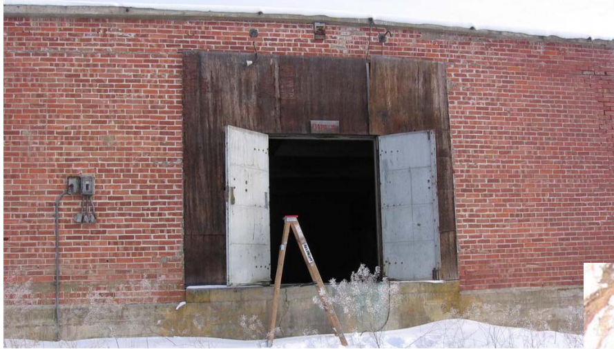
Photo No. 5: Typical front view of bunkers (February 4, 2008).
