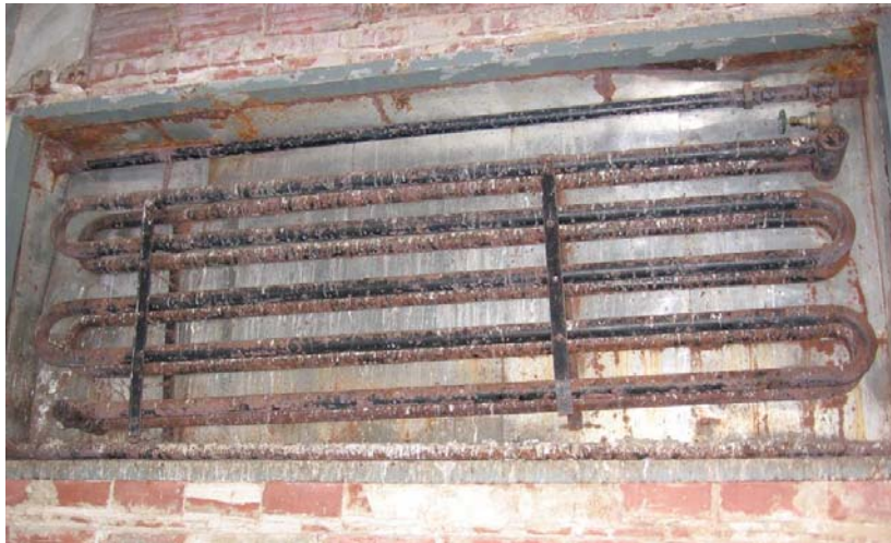
Photo No. 8: Piping inside bunker walls with asbestos pipe wrap still present (February 4, 2008).
