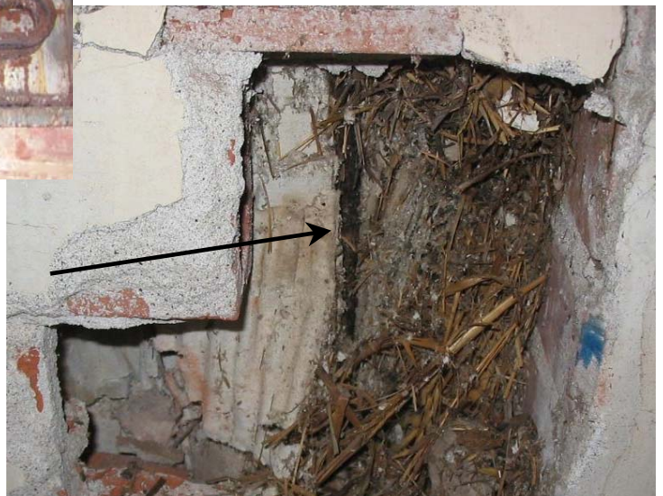
Photo No. 7: Example of pipes used for heating interiors of bunkers. Asbestos pipe-wrap has already been removed (February 4, 2008).
